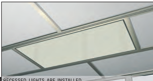
13 RECESSED LIGHTS ARE INSTALLED
